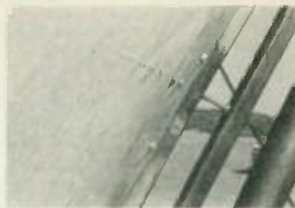
FIG. 7—SPHERICAL SHAPE is created by gently shaping the contour with 10x24 adjusting screws spread from center of reflector surface outward along spokes. Actual tweaking is done with a measuring device extended from radius point stretched taut to antenna surface.
